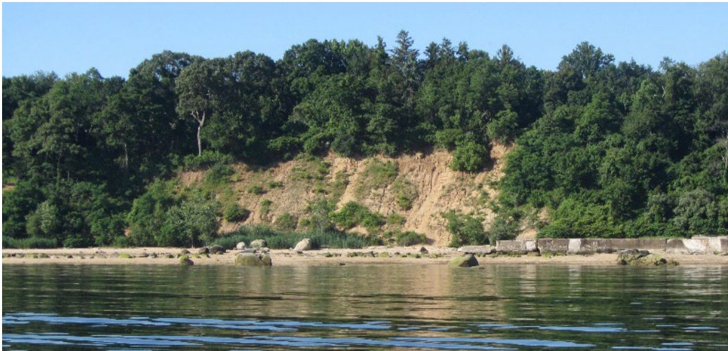
Washouts along the west shore (photo by Carol DiPaolo, 6/29/22)
