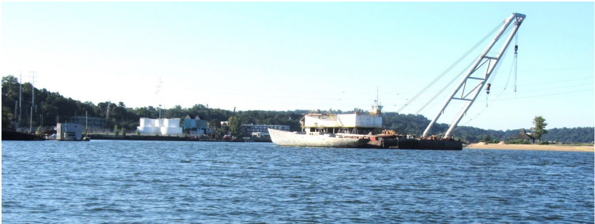
South view of Hempstead Harbor and east shore with National Grid property to the left and Gladsky Marine crane to the right (photo by Carol DiPaolo, 8/3/22)
